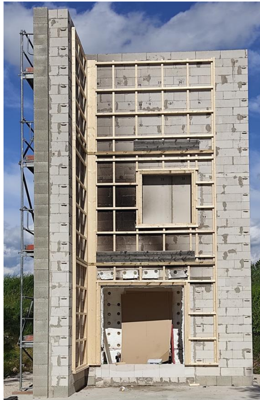
Figure 4.2. Specimen without the timber cladding at ÉMI's laboratory. Additional cavity barriers and additional support for the cladding. Open cavity at the top.
