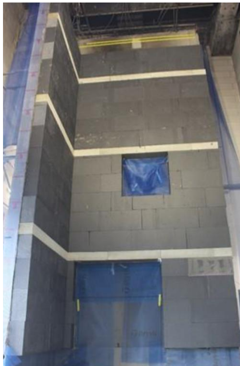
Figure 4.5. Specimen is under construction at the laboratory of MFPA.
