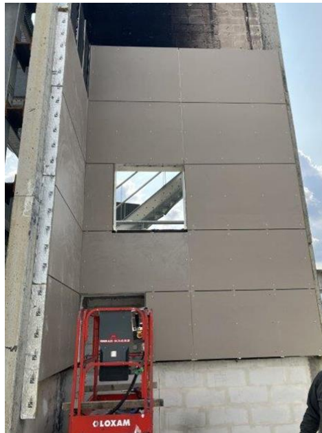
Figure 4.8. The tested Fiber cement façade at the laboratory of Efectis
